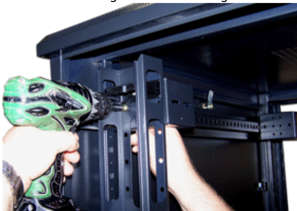
Installing the cable manager
